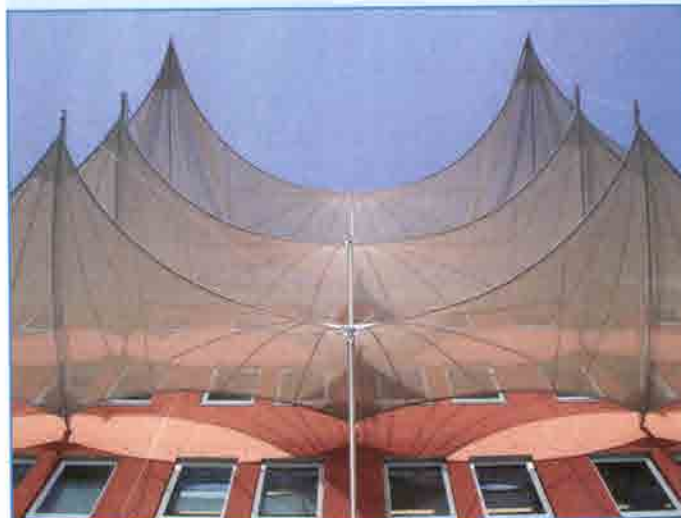
CHARLEROI / Gosselies. EOLE. © IGBETEC.
