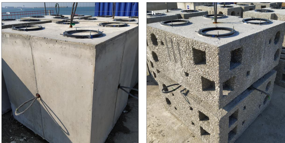
Figure. 1. Dyke modules deployed during the MARINEFF project: a: classic module; b: Eco-engineering module.
