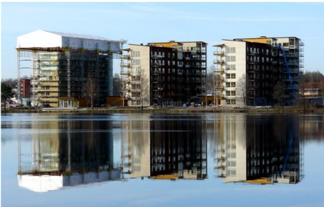
Figure 6. Limnologen, 3 of 4 buildings. Photo by K. Jarnerö, April 2008
