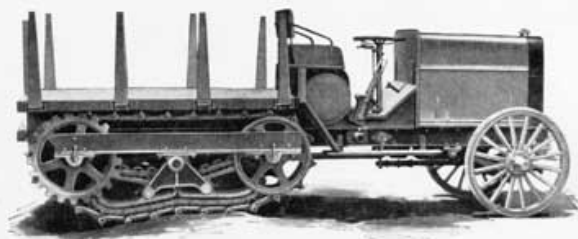
The Linn Tractor passing over an unevenness in the road, showing the Self-Laying Track always clinging to the ground. It travels in the field equally as well as on the highway Plate Four
