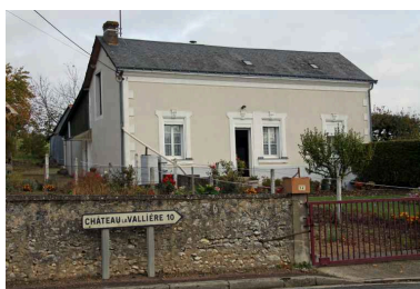
12, rue Principale. Phot. Jean-Baptiste Darrasse IVR52_20087202441NUCA
