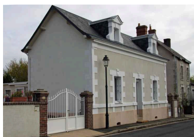
10, rue Principale. Phot. Jean-Baptiste Darrasse IVR52_20087202440NUCA
