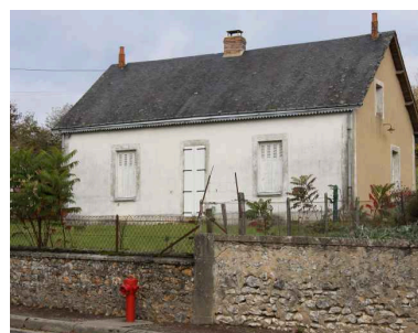
14, rue Principale. Phot. Jean-Baptiste Darrasse IVR52_20087202442NUCA
