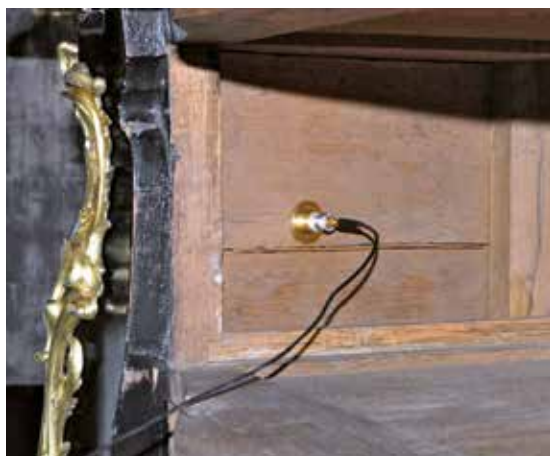
Fig. 1. An AE sensor located close to the tip of an existing crack at the wall of the commode which is the area most at risk of climate-induced fracturing
