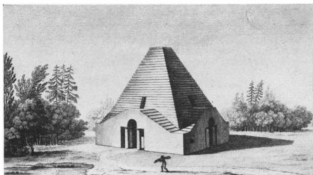
FIG. 167. First house of the lumbermen—Atelier des bûcherons.
