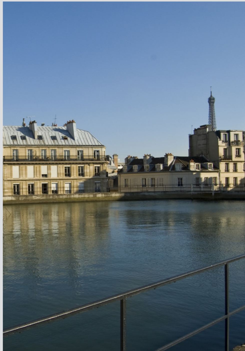
Reservoir eau non potable Paris
