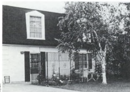
Target hardening by using screens to improve building security increases the difficulty of illegal access.
