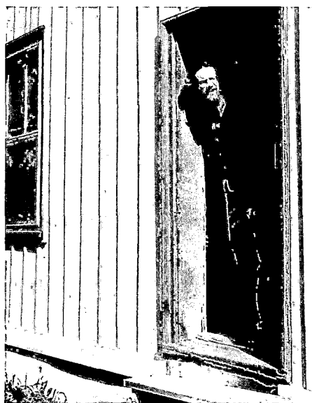
Under a grey stucco exterior that had been applied at some point during the life of the house, Hepburn found and restored the original board and batten siding.
