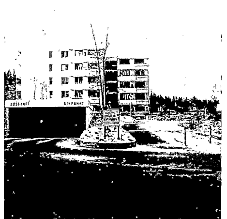
Vehicular traffic is controlled by barrier posts to keep cars off residential lanes, and underground parking. The entrance/exit ramp for the garage is located on the left.
