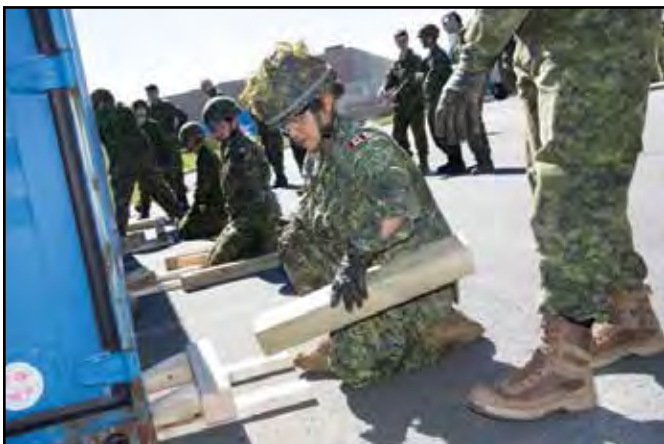
Basic LUSAR training in Halifax Sept. 21 to 23, 2018. Members of the LUSAR team practice cribbing.
