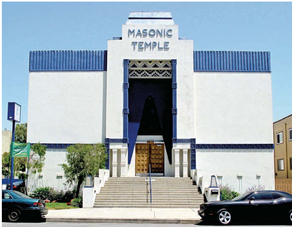
Fig. 44 : Temple North Hollywood, Californie. Robert Stacy-Judd & John Aleck Murrey architectes, 1949 Source : https://commons.wikimedia.org/wiki/File:Masonic_Temple,_North_Hollywood,_CA.jpg/
