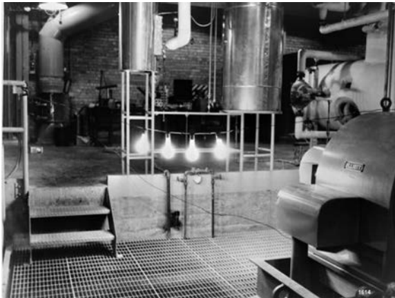
FIG. 2.4. Light bulbs at Idaho Falls, USA powered by steam generated by a nuclear reactor (reproduced with permission courtesy of the Idaho National Laboratory, USA).
