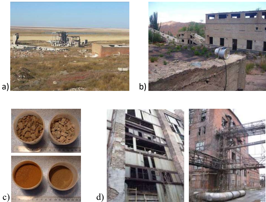
FIG. 9.4. Examples of the remaining infrastructure at former uranium mill sites: (a) former uranium mill site, Zaozerniy, Kazakhstan (2015); (b) former mill site, Kadji-Say, Kyrgyzstan (2007); (c) uranium raw materials sieved from the contaminated temporary raw material storage area at the former mill site, Prydniprovskyy Chemical Plant, Ukraine (2016); (d) current state of the former uranium extraction facilities at the Prydniprovskyy Chemical Plant (photographs taken by O. Voitsekhovych, Ukrainian Hydrometeorological Institute).
