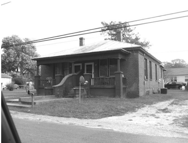
Double House, 25715 Nottoway Street, West Petersburg (026-5128) from northwest
