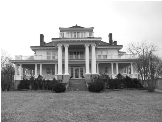
Gatewood (026-5162), view from northwest
