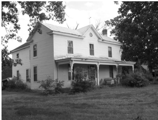
Leonard House (026-5085), view from southwest
