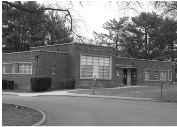
Dinwiddie County Health Department (026-5130), view from the southeast
