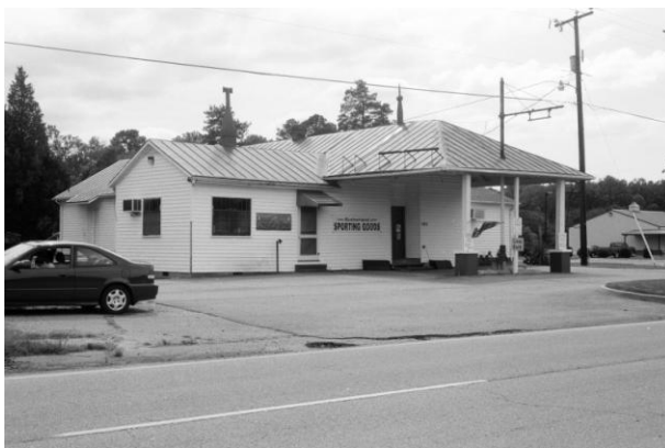
Alban Sutherland Store (026-5089), view from northeast
