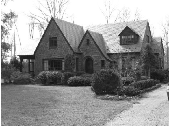
Hargrave House (026-5166), view from east
