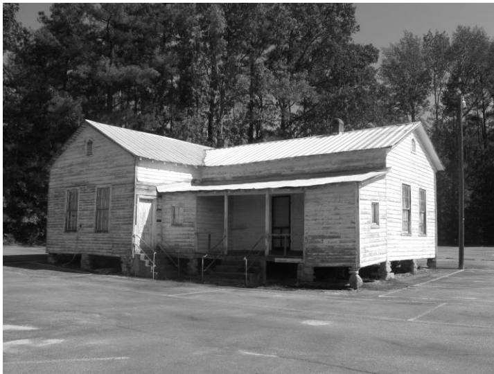
Rocky Branch School (026-5114), view from south
