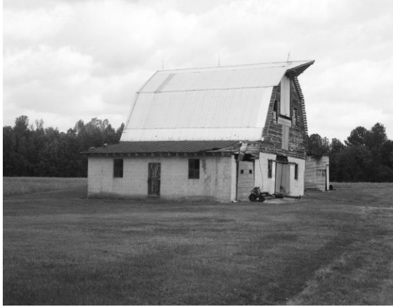
Barn, 5021 Midway Road (026-5119), view from southwest
