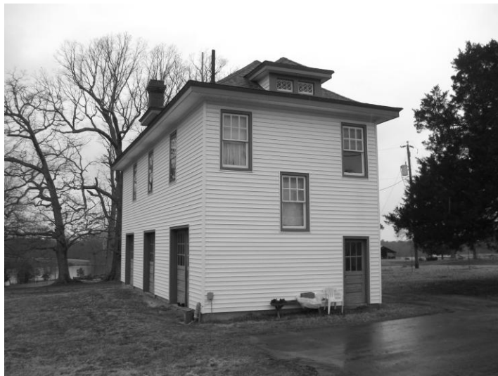
Garage, Gatewood (026-5162), view from east
