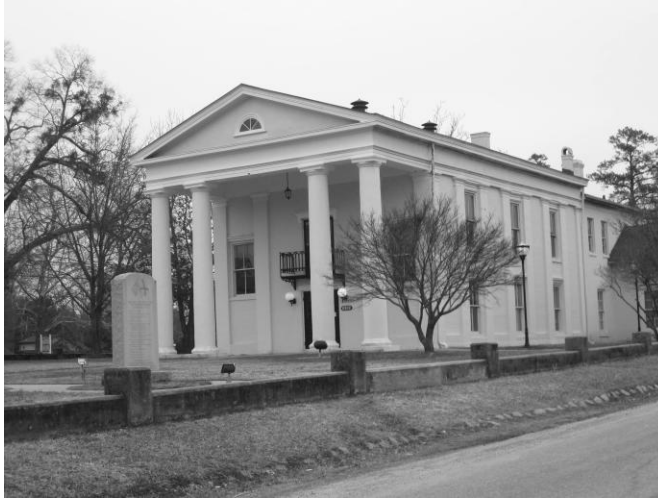
Dinwiddie County Courthouse (026-0004), view from southwest
