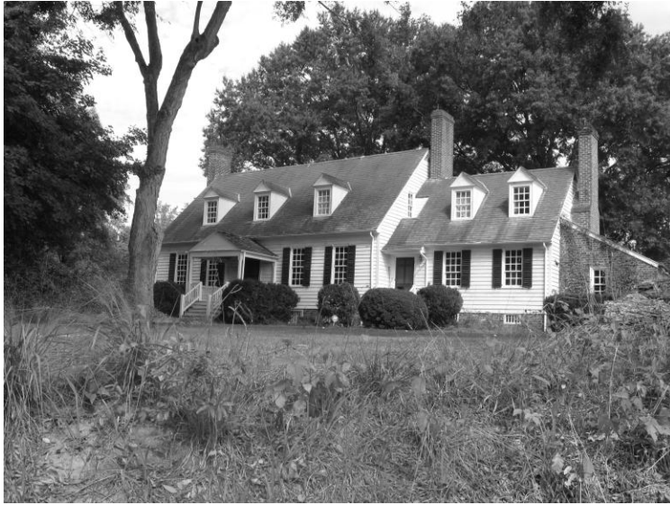
Burlington (026-0001), view from southeast
