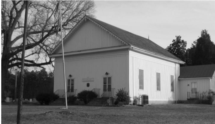
Butterwood Methodist Church (026-0111), view from northwest
