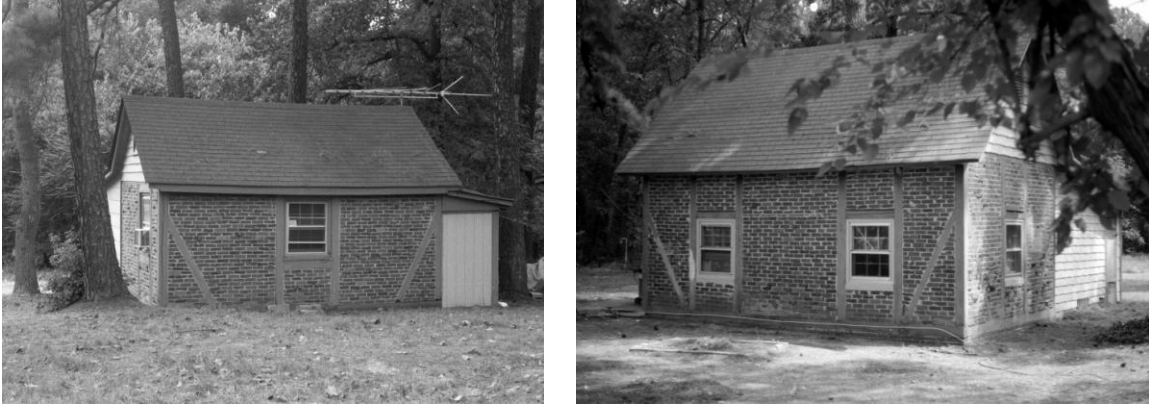
Ye Blue Tartane Motor Court (026-5081), single-room unit from east (left) and two-room unit from west (right)
