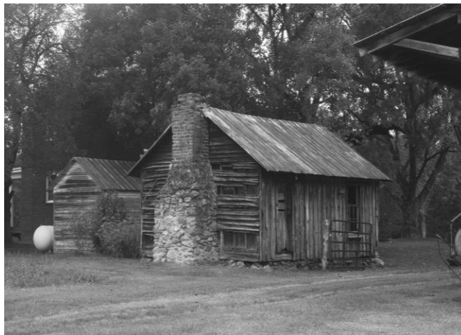
Kitchen at 5021 Midway Road (026-5119), view from northeast
