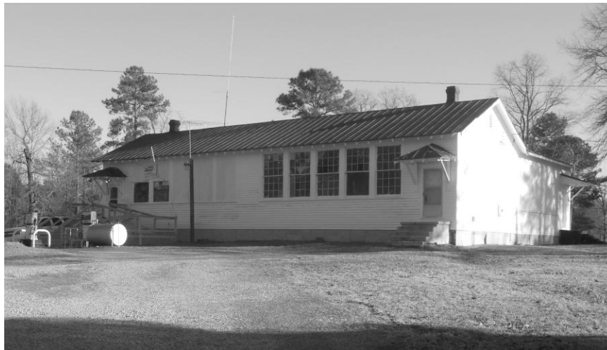
Masontown School (026-5175), view from northwest
