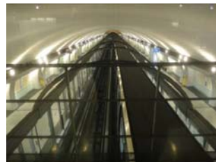
Figure 8 – Ligne 14 / MP 89 ca – Station Olympiades
