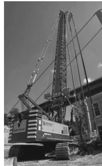
Figure 8. Diaphragm Wall Machine, Hydrofraise-Cutter
