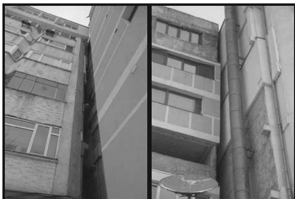
Figure 3. Photos showing on site displacements
