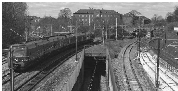
Figure 2. Picture taken prior to project start up showing the 5 railway lines.
