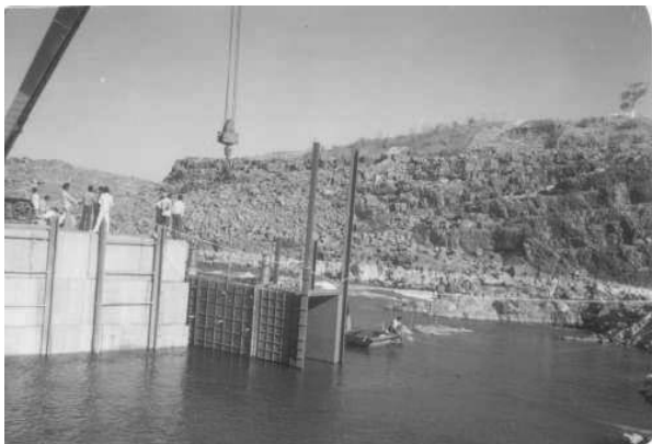
4.10 Masonry Works above water level.
