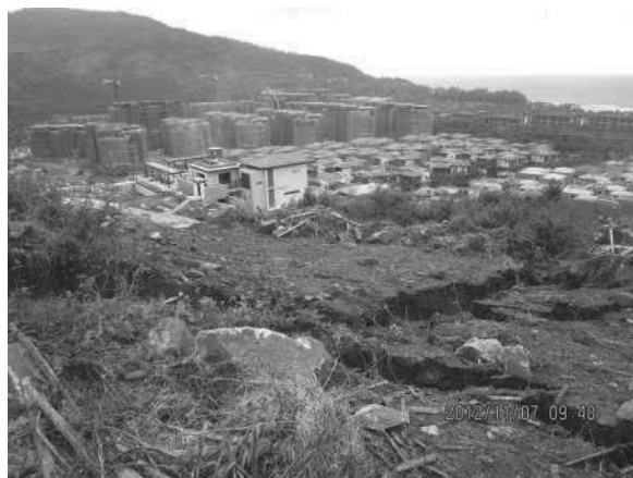
Figure 5. Failure of the sliding slope during a heavy rainfall on November 4, 2012.
