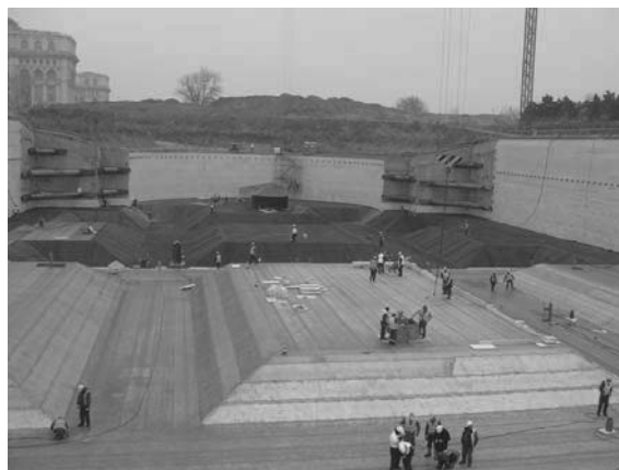
Figure 9. Lead waterproofing
