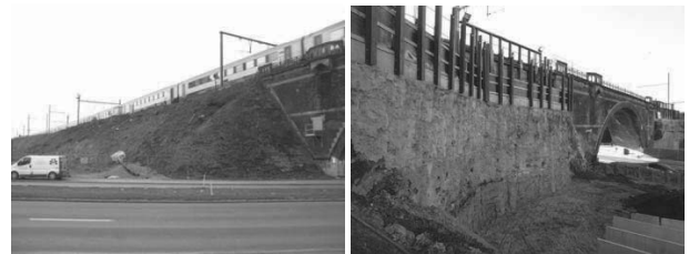
Figure 1. Picture of initial situation (left) and picture of the jet grout wall after excavation (right).
