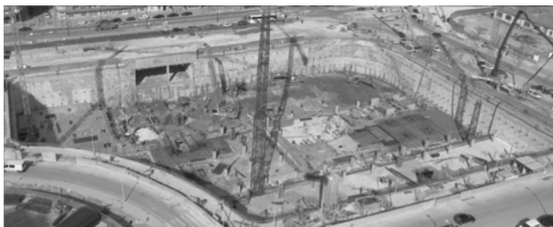
Figure 13. General view of the jobsite at design excavation level.
