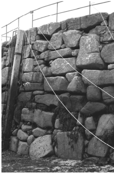
Figure 4. Wall at Mousehole, Cornwall, containing of large blocks.
