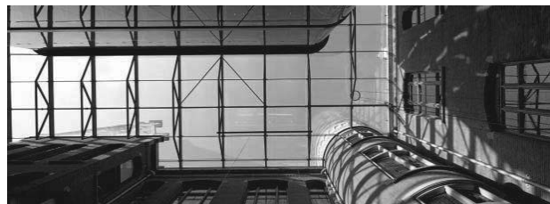
Figure 15. Finished construction – atrium new-old
