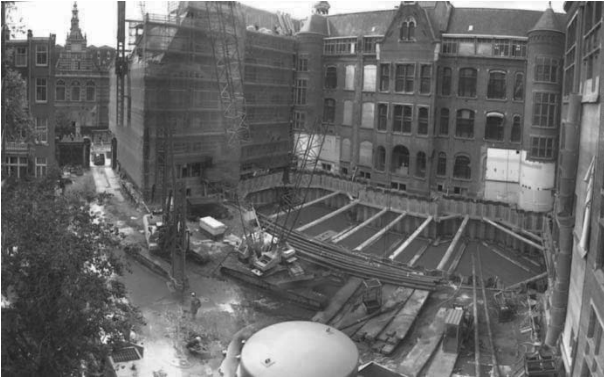
Figure 8 Overview building pit (at the time of incident)
