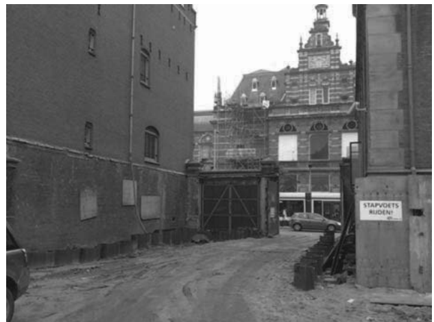
Figure 12. Building pit at PP44 before incident
