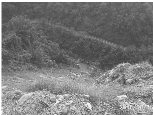
Figure 12. Downhill slope of Mt. Ali road section at Mileage 39Km.
