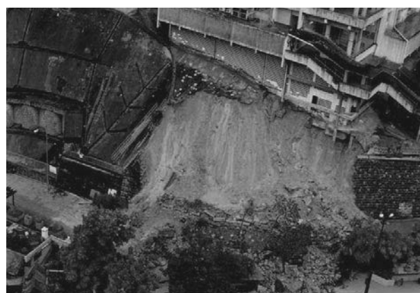
Figure 1: The Kwun Lung Lau Landslide in July 1994
