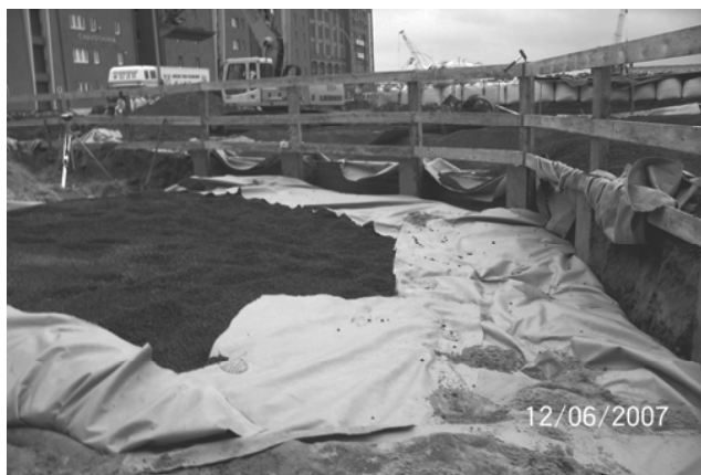
Figure 5: Placing of expanded clay
