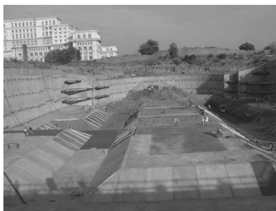
Figure 8. Final stage of excavation
