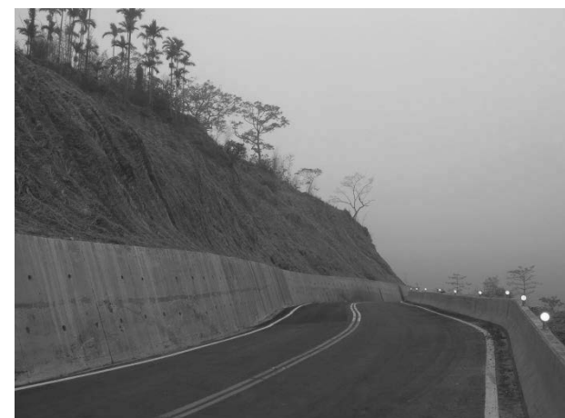
Figure 10. Completion of upslope remedial works at Mileage 39Km.
