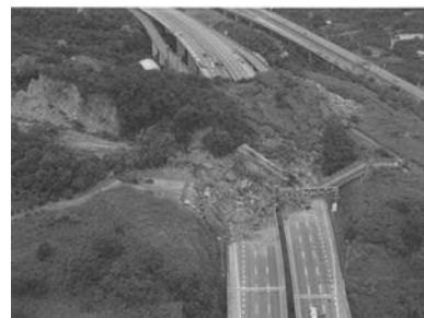
Figure 1. National Highway No. 3 at 3.1k accident
