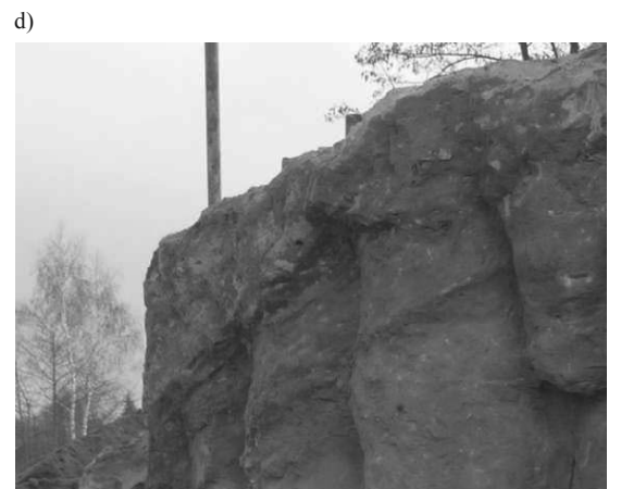
Figure 4. Different shapes of excavated jet grouting columns (photos: J. Bzówka, and K. Wanik).
