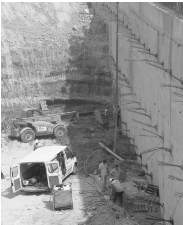
Figure 14. Execution of acceptance tests in El Corte Ingles
