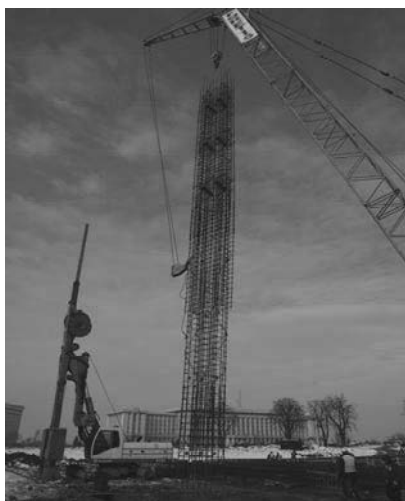
Figure 6. Installing the reinforcement cage of the diaphragm wall
