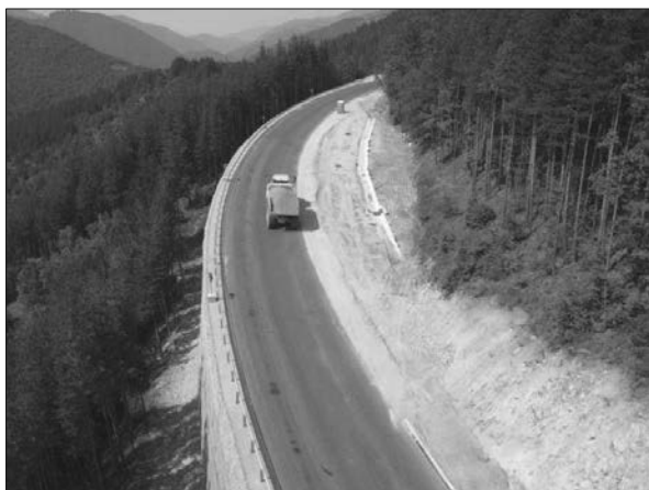
Figure 9. Top view of a completed GRS-wall.
