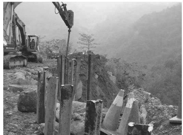
Figure 9. Emergency repair of the road section due to Typhoon Talim.
