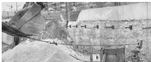
Figure 16. Removing an anchor unit with a force of 50-150 kN.
