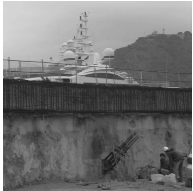
Figure 10. Investigation test in trial SBMA anchor in the port zone.
