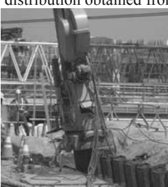
Photo 2. Overall view of installation work
