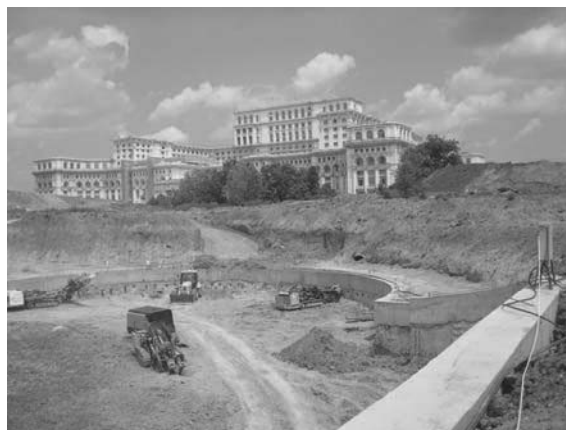
Figure 7. Installation of the first level of anchors
