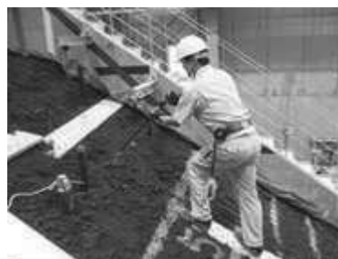
Photo 1. Installation of MPS
