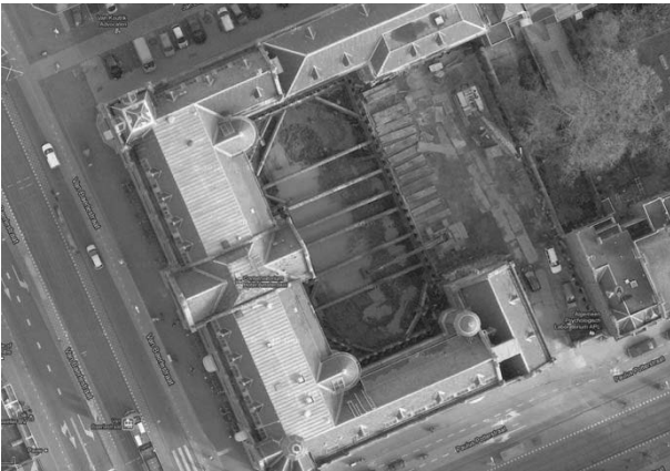
Figure 9. Top view building pit (at the time of incident; © Google)
