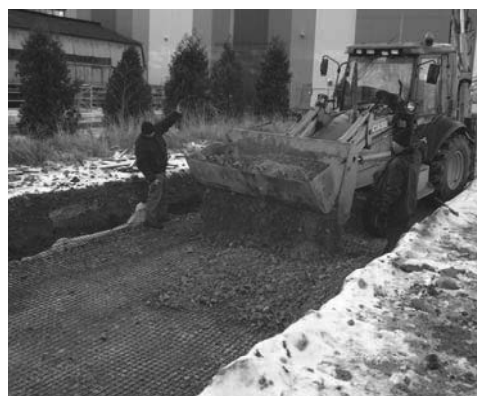
Figure 5. Construction of the experimental reinforced crushed stone pad
