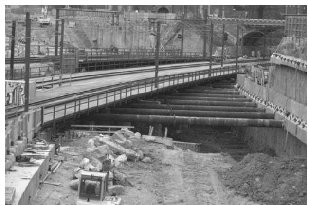
Figure 15. Picture of the railway crossing, December 2012.
