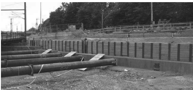
Figure 9. Encastered soldier pile wall.
