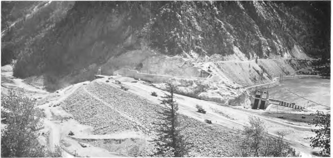
TERZAGHI DAM DURING CONSTRUCTION
