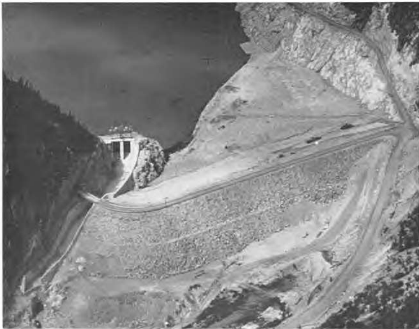
TERZAGHI DAM—CONSTRUCTION COMPLETED AND RESERVOIR FILLING
