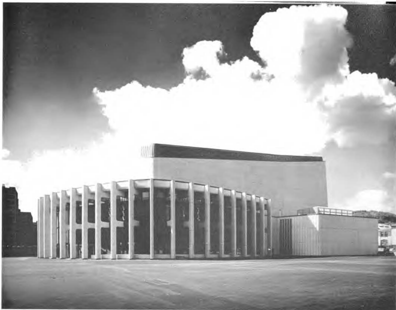
EXTERIOR VIEW, PLACE DES ARTS, MONTREAL—SITE OF THE SIXTH INTERNATIONAL CONFERENCE—8-15 SEPTEMBER 1965.
