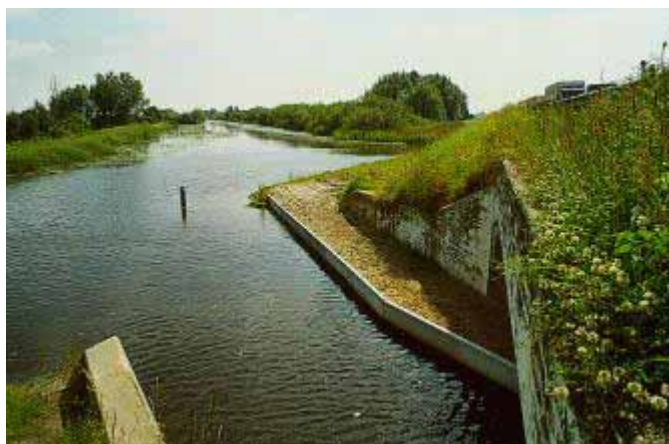
Figure 2 : Adapted bridge under highway in The Netherlands, for amphibian, mustelidae, insects (Photo by Hans Bekker)
