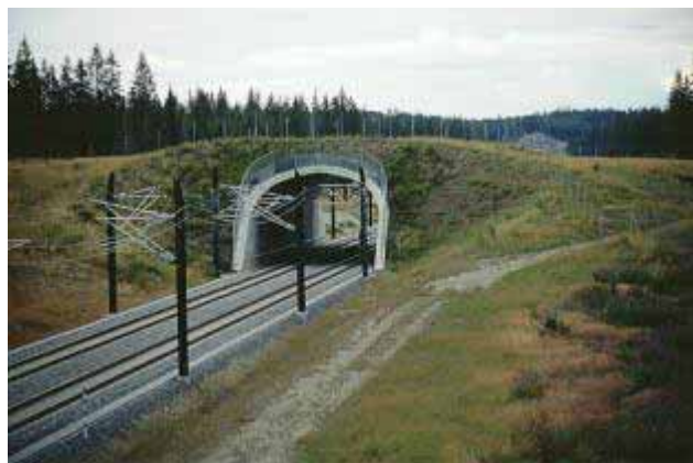
Figure 3 : overpass in Norway over train, to use by small and large animals (Photo by B. Iuell)
