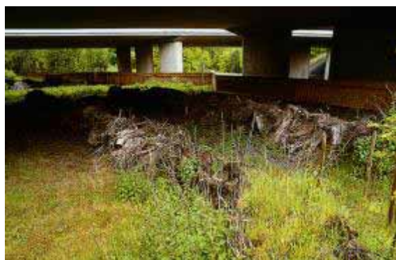
Figure 5 : Tree stumps as guidance for amphibians, insects and small mammals under a viaduct (Photo by Henry Cormont)
