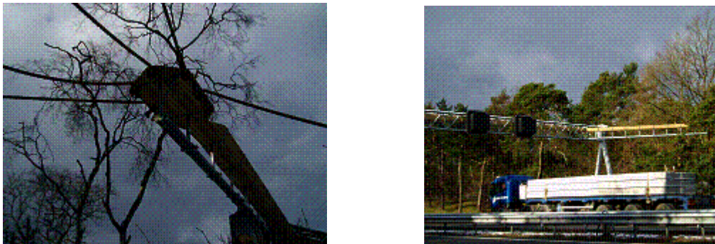
Figure 6 : Innovation: adaptation of a gantry for traffic information for joint use by squirrels and pine marten in the Netherlands (Photos by Hans Bekker)
