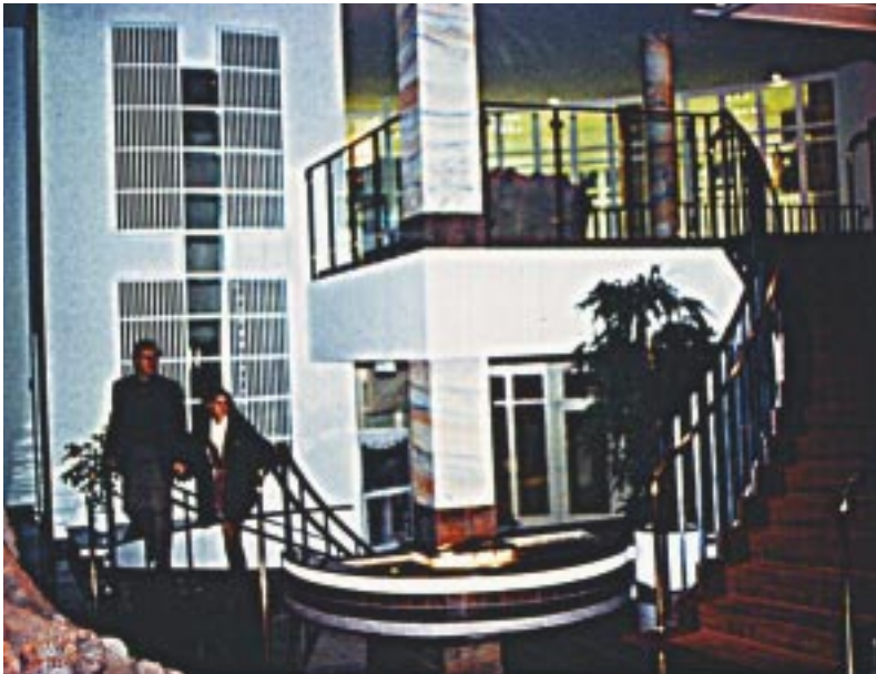
Above the stairs, on the left, in the hotel, the grills on the right-hand side are supply air units, while the grills on the left-hand side are only decorative and serve to maintain the architect's balanced design.
