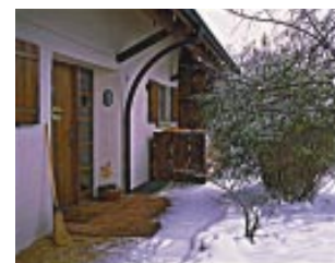
The family home at Rünenberg. The air-to-water heat pump is installed in the cellar. Tap water is prepared separately by a second small air-to-water heat pump.
