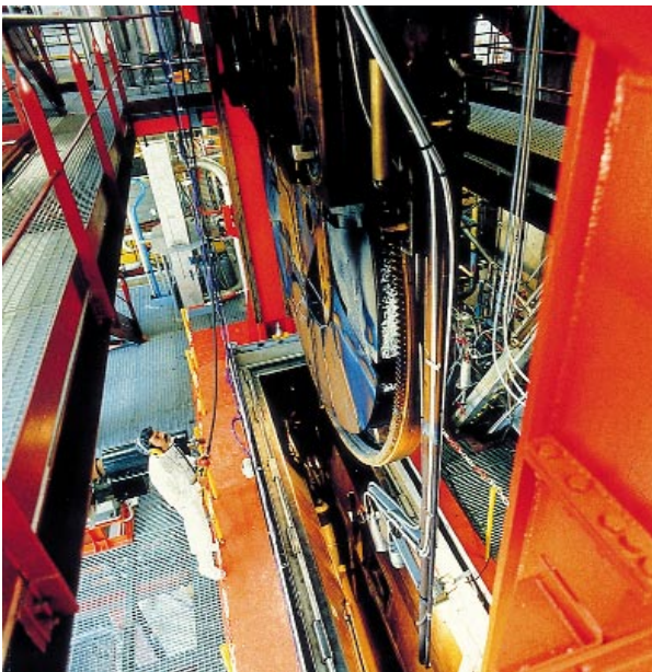
Usine UP 3 : dissolvant (lors de la construction)
