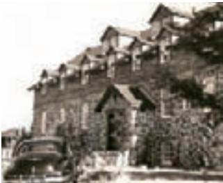
31 The Nymark Lodge at the foot of the slopes (around 1950)
