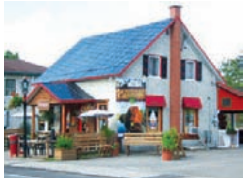
17 House with blue roof, 269, Principale
